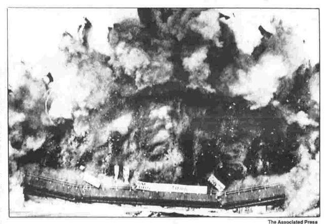
THAR SHE BLOWS — A farm access bridge in Kegworth, England is blown up to make way for a new junction. Traffic was diverted as the bridge was demolished with 77 pounds of ex-
